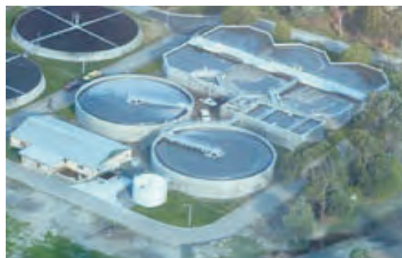
Figure 8.7 An aerial view of a sewage plant
